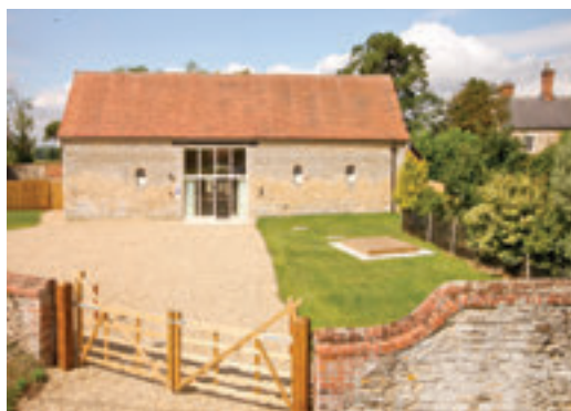
Manor Barn Walcot
