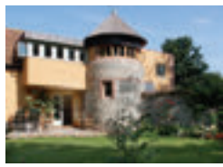
Rectory Cottage Wilby near Old Buckenham
