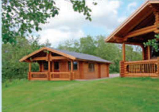
Cabin 10, Felmoor Park Felmoor Park
