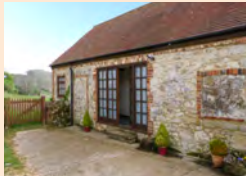
Stable Cottage Gatcombe
